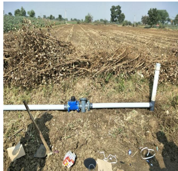
Installation of Water Meters at Demonstration Plot in Madana
