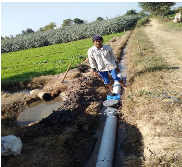
Installation of Water Meters at Demonstration Plot in Madana
